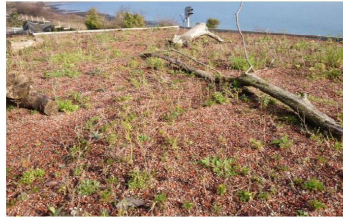
Functional inaccessible Brown roof systems
